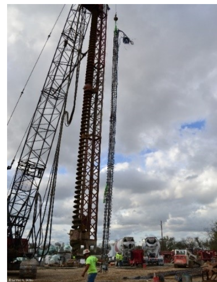
Figure 1.4.8 – Energy pile being installed
