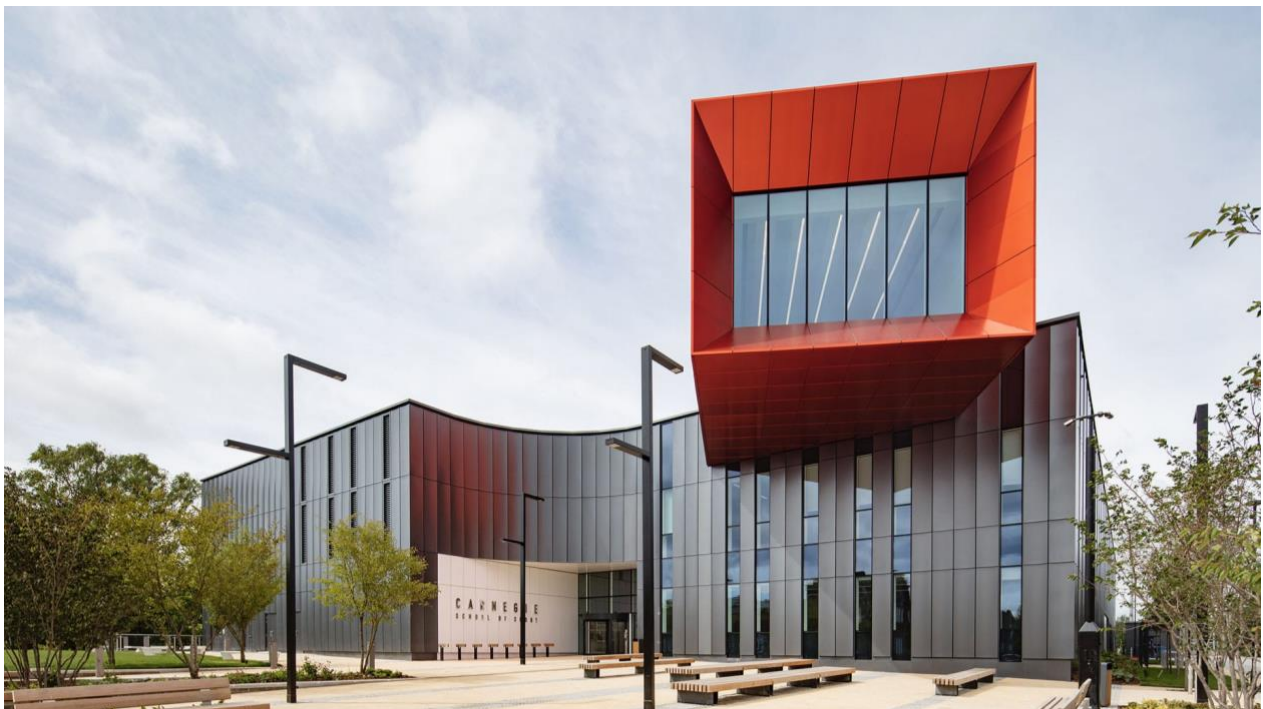
New £45M state-of-the-art building for the Carnegie School of Sport (Opened May 2020)
