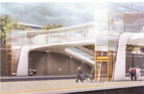
Figure 3: Futura FRP Station Footbridge, reproduced with kind permission from Marks Barfield Architects and COWI
