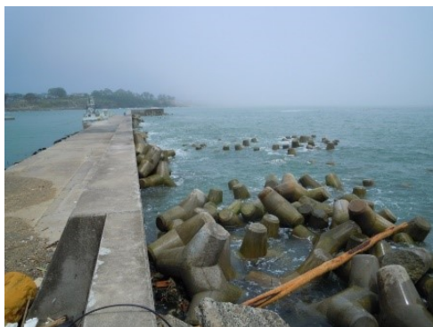
Figure 1. Displacement of artificial armour units after 2011 Tsunami
