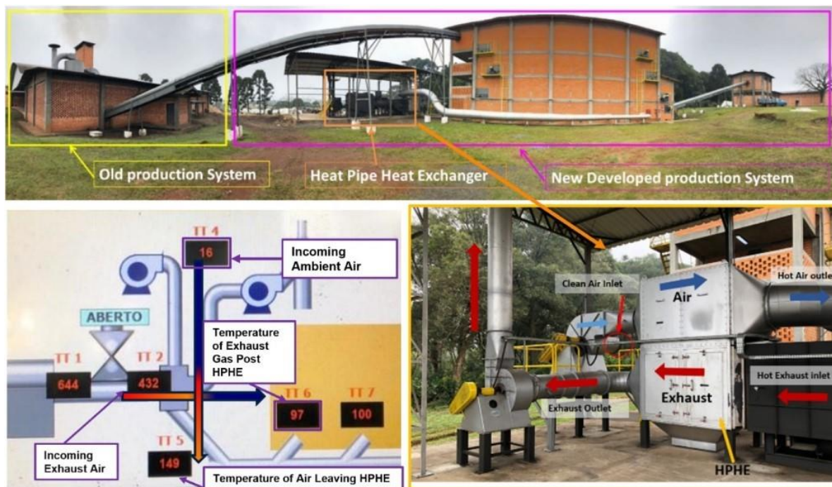
Figure 1: The installed Heat Pipe Based Production Line at Ervateira
