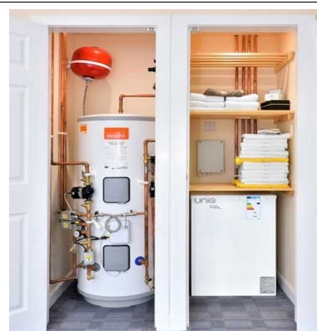
Figure 2. Sunamp heat battery (right), showing space saved compared to traditional hot water cylinder (left).
